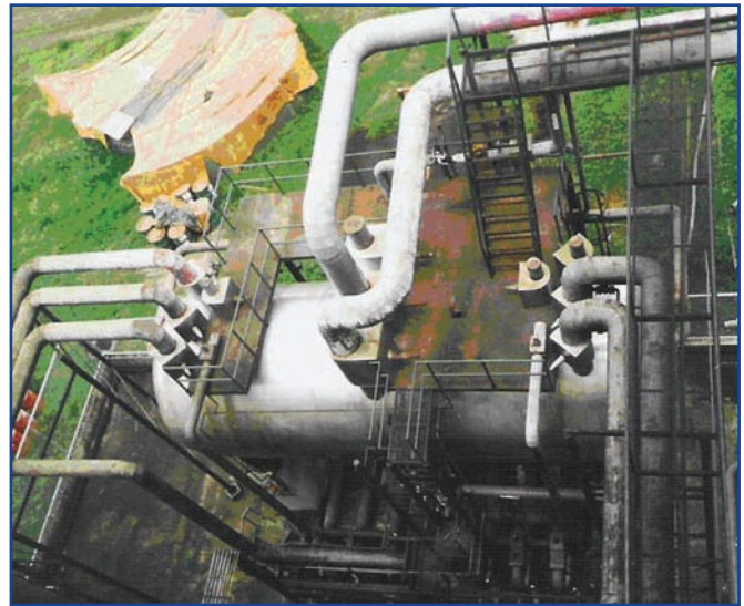
Left: Inflating clamp-on cooling panels. Right: Top of existing 5275 kW (1,500 ton) \text{NH}_3 separator to be retrofitted to 12 309 kW (3,500 ton) separator.
