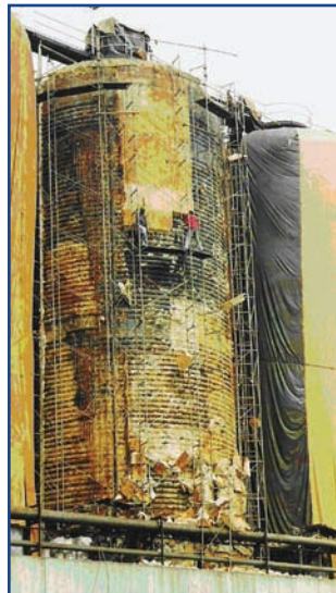
Left: Dismantling of \text{NH}_3 cooling jackets. Right: Installation of laser-welded cooling panel with heat transfer paste.
