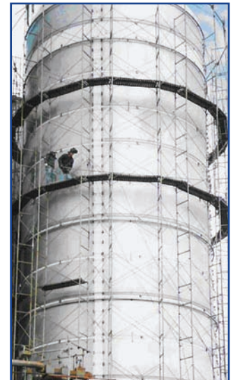
Left: Dismantling of \text{NH}_3 cooling jackets. Right: Installation of laser-welded cooling panel with heat transfer paste.
