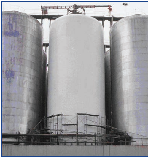
Retrofitted conical tank with laser cooling panel.
